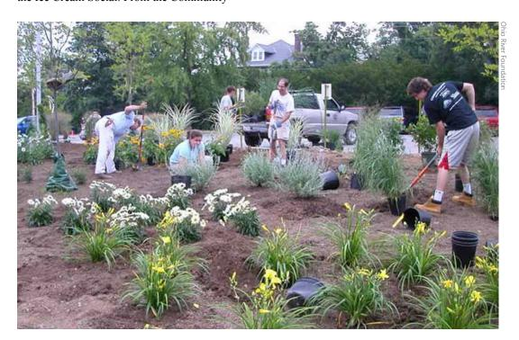
Rain gardens collect stormwater from impervious surfaces reducing the amount of water flowing into storm drains.
